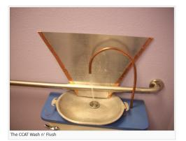
A toilet modification that allows users to save water by utilizing the wastewater from handwashing to flush the toilet.
